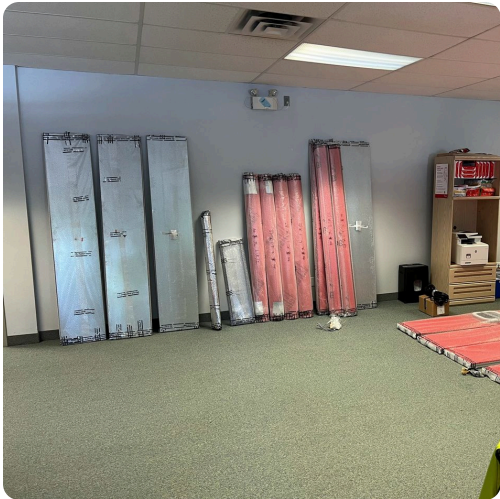
01 Panels arrive flat and wrapped.
